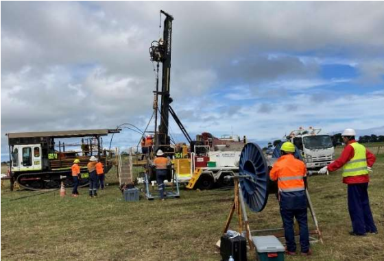
Figure 3 Fiber optic installation work at Otway site
