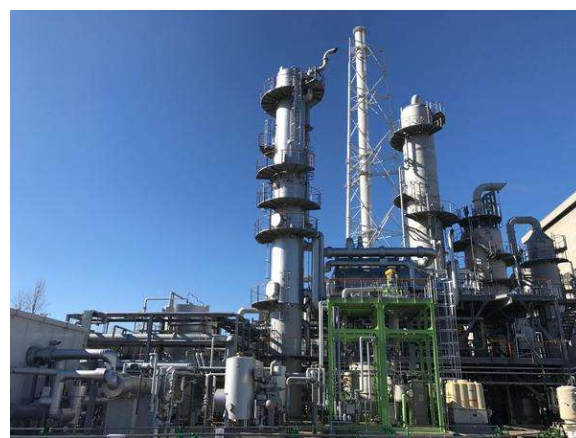
Fig. 1. Equipment of energy-saving CO 2 absorption process ESCAP ® at Niihama Nishi power station, Sumitomo Joint Electric Power Co., Ltd.
