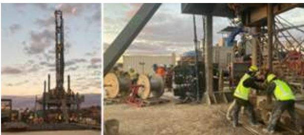
Figure 4 Fiber optic installation at the southern Perth site, Australia
