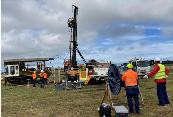
Figure 3 Fiber optic installation work at Otway site
