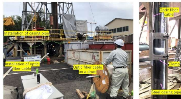
Figure 1 Fiber optic installation work at a site in Japan
